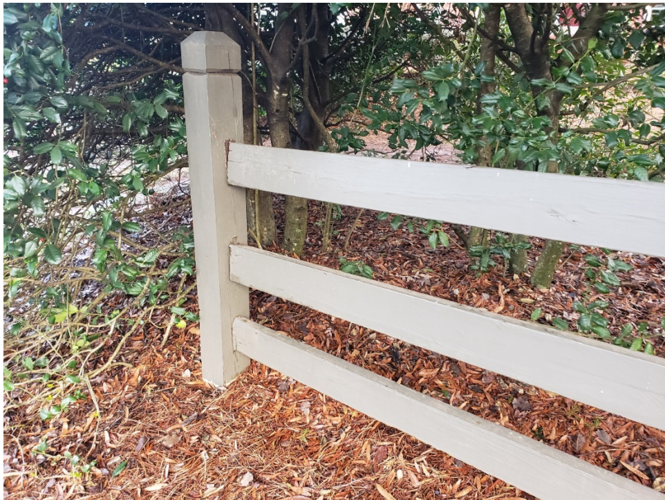
6. View of typical entry fence. Note the rotating horizontal members.
