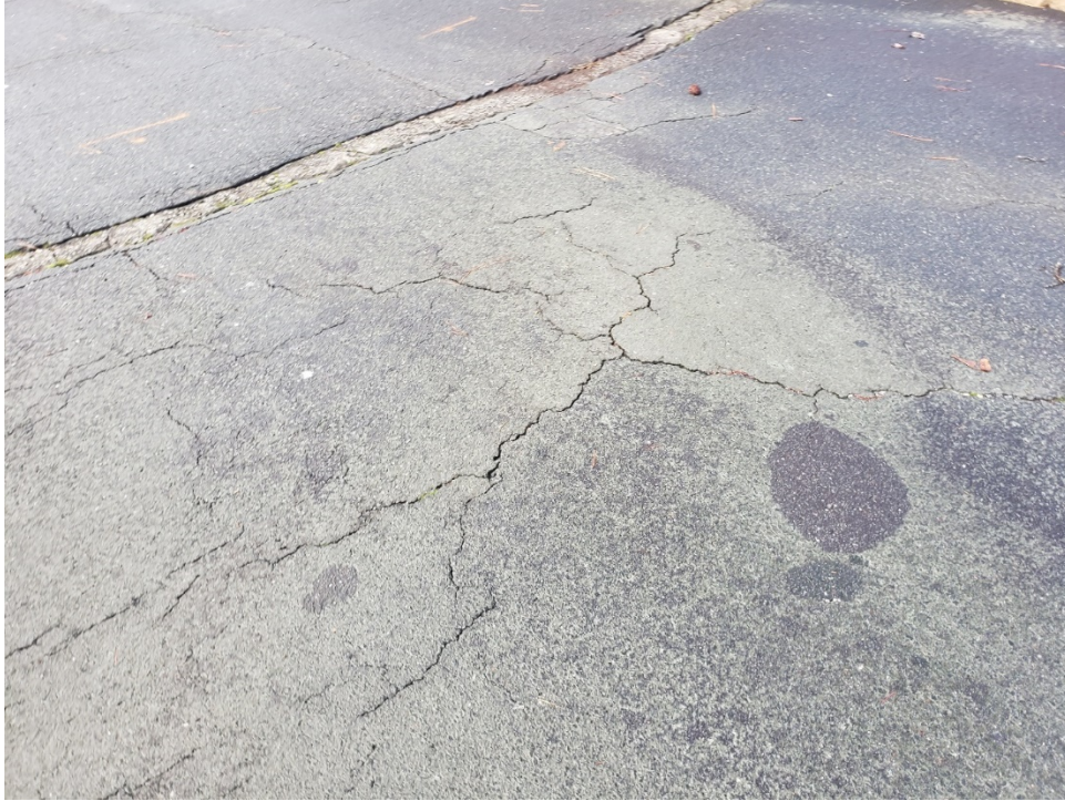
1. View of linear cracks at the amenity area parking lot.
