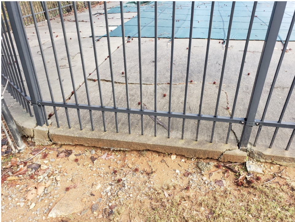
10. View of voids beneath the concrete pool deck as a result of poor drainage.
