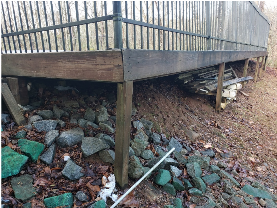
18. View of failing section of the wood-framed pool deck that should be replaced.
