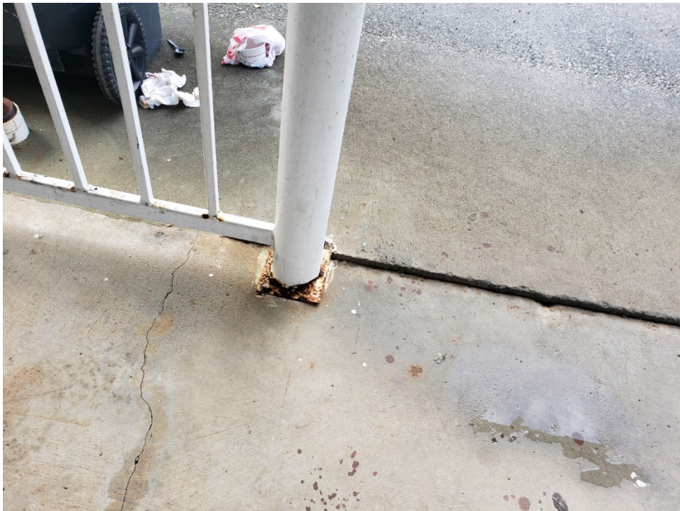
26. View of typical corroded pavilion column at the pool house.
