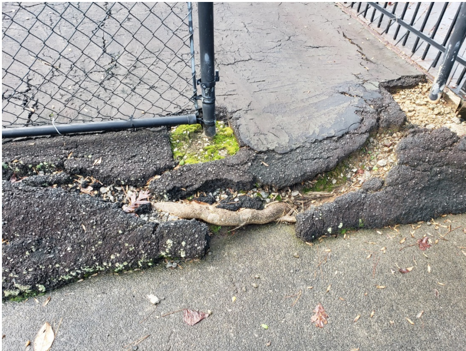
8. View of tree roots damaging a section of the basketball court.
