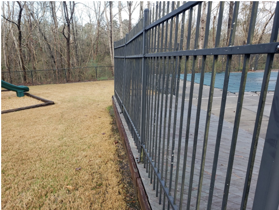
14. View of leaning section of the pool fence.
