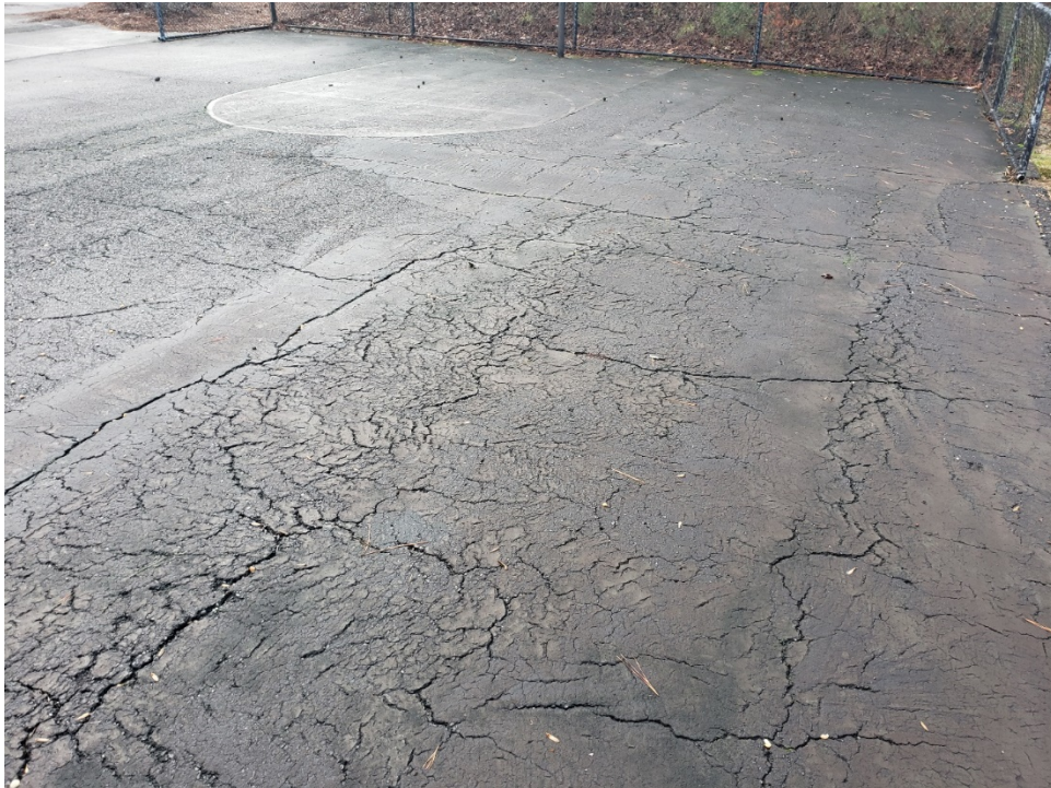
20. View of multiple cracks and settled sections of the basketball court.
