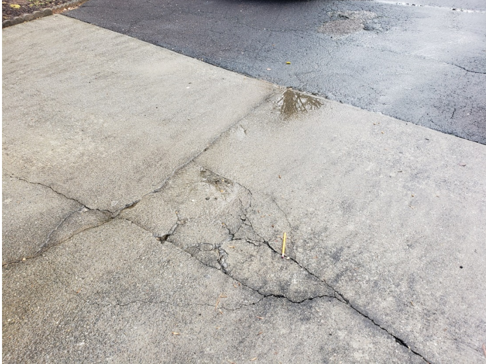
3. View of cracked and settled section of the concrete.
