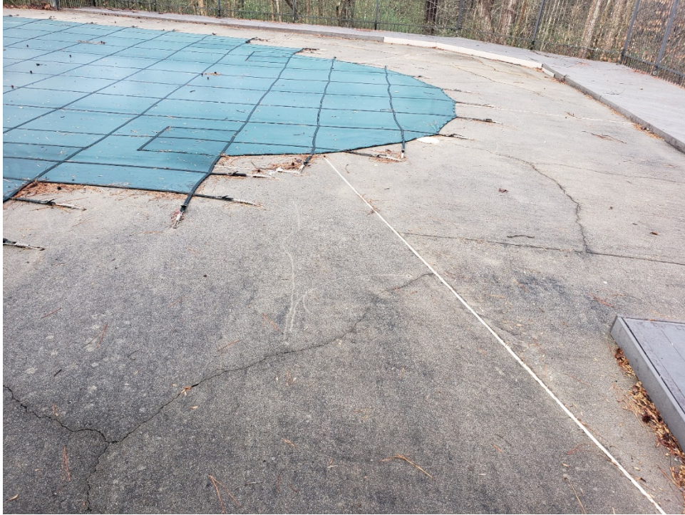
13. View of typical linear cracks at the pool deck.
