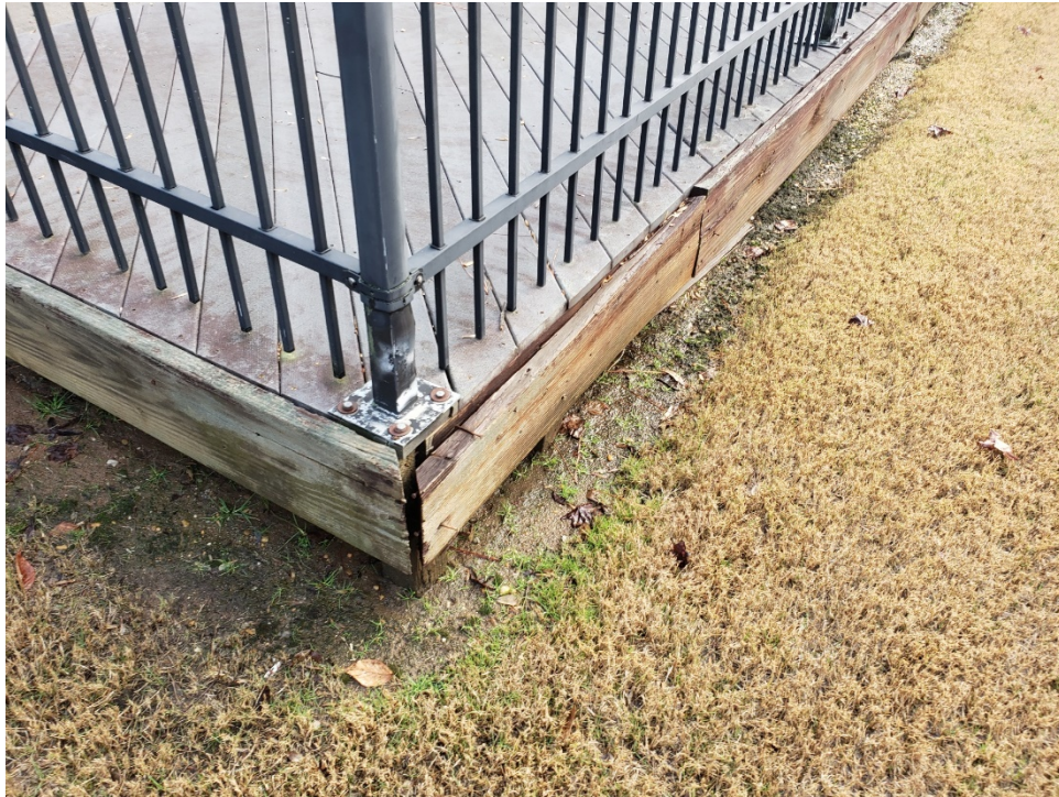
17. View of deteriorated band at the wood-framed pool deck.
