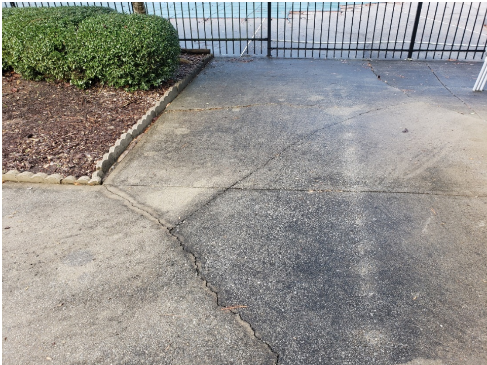
4. View of cracked and settled section of the concrete.
