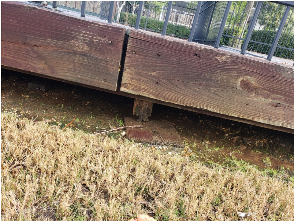
16. View of deteriorated band and 4x4 column at a section of the wood-framed pool deck.
