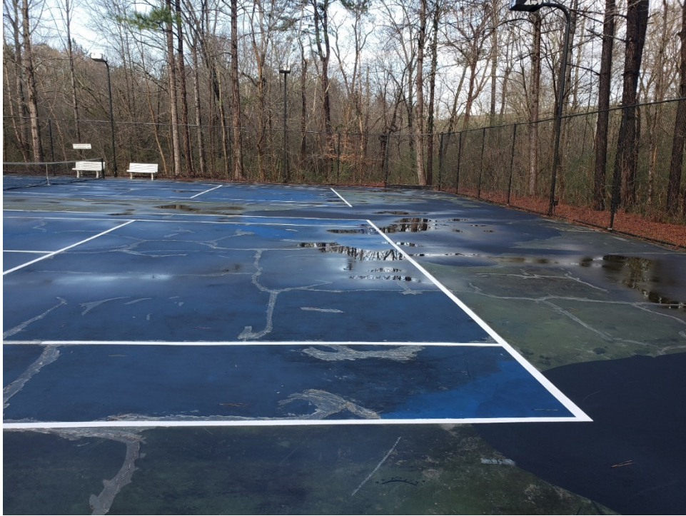
19. View of ponding water and cracks at the tennis courts.
