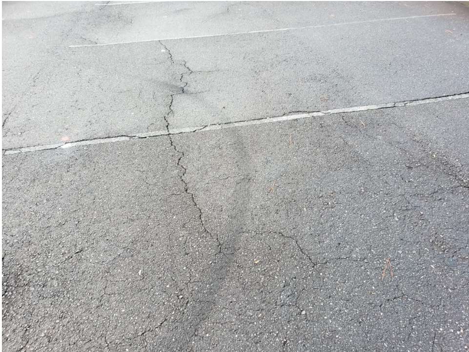
2. View of linear cracks at the amenity area parking lot.
