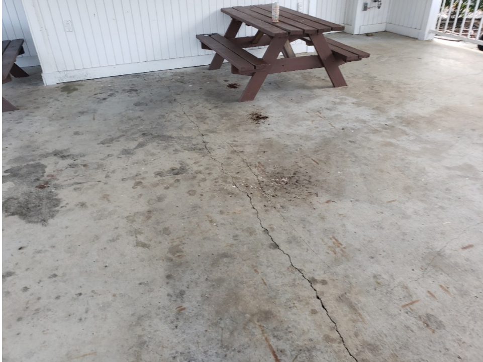
25. View of typical linear crack at the pool house concrete slab.
