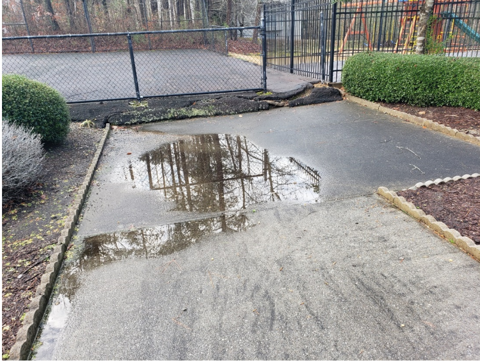
9. View of ponding water between the amenity area concrete and basketball court.
