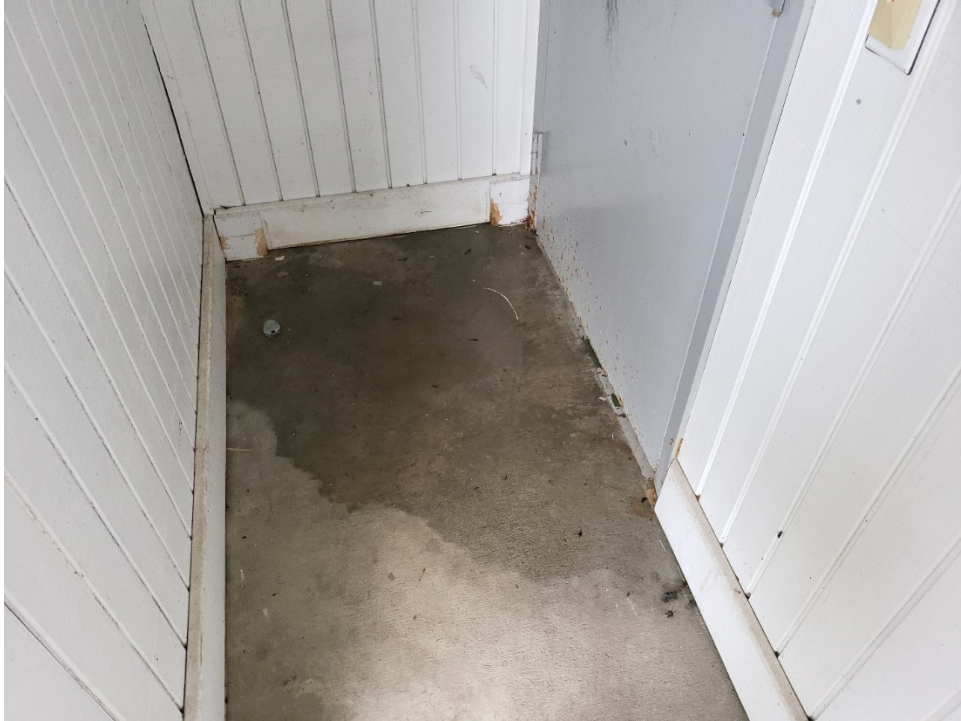
27. View of ponding water in front of the restroom doors.
