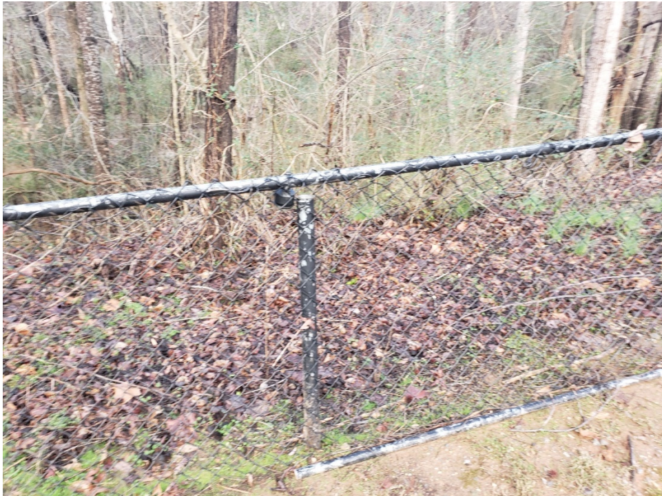
12. View of typical section of chain link fence that has chipped paint and is damaged.
